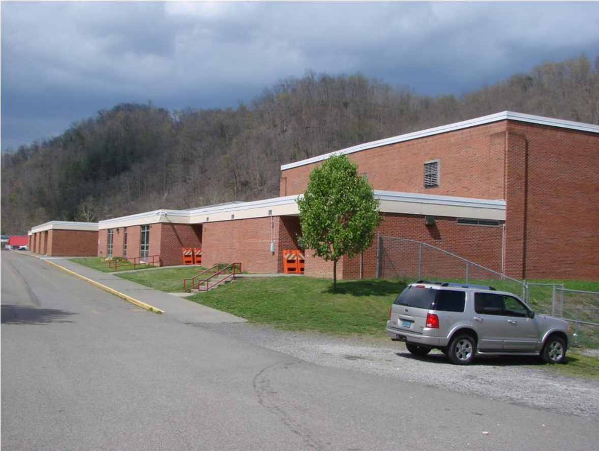
Main School Structure
