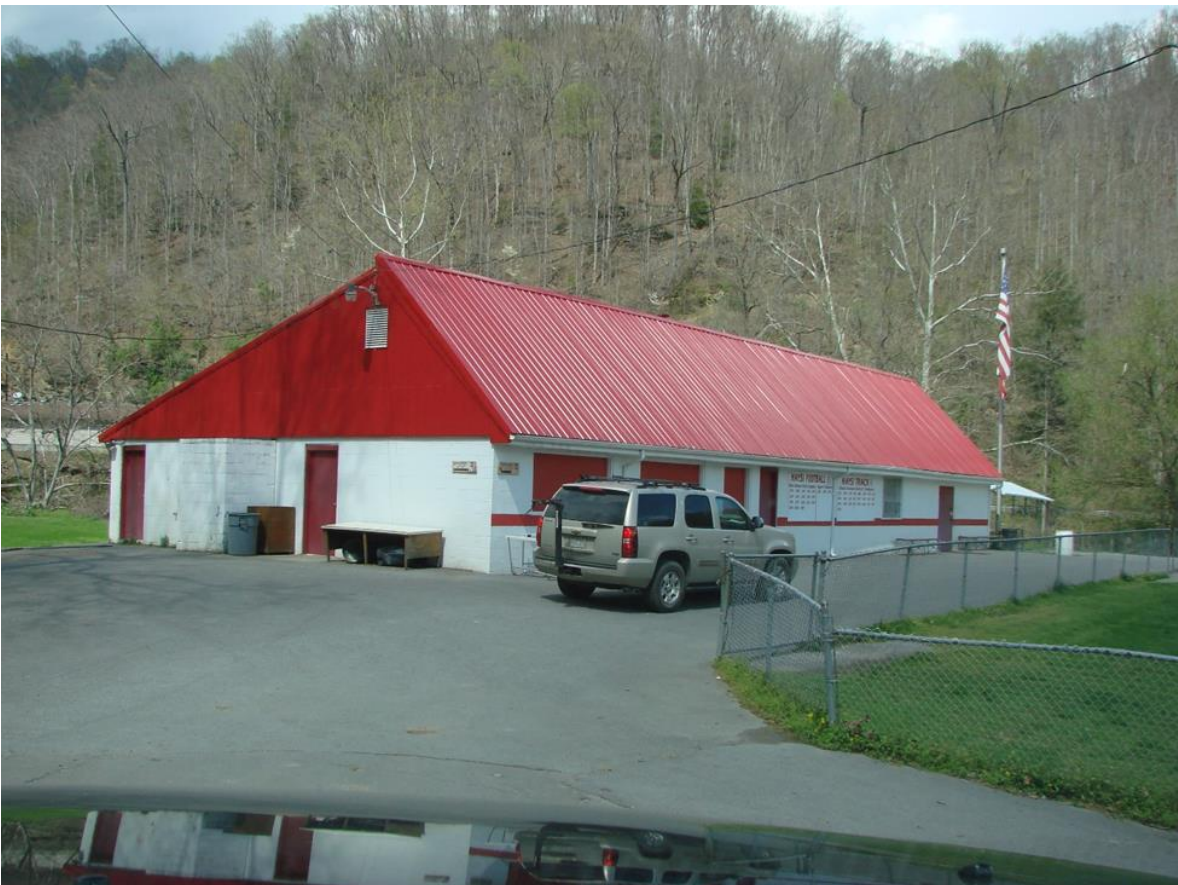
Fieldhouse and Pump Station
